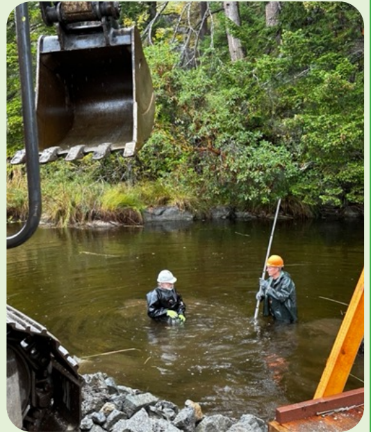
2 - Jim and Dave preparing the level base for the lock block to rest on. The depth had to be within a few cms.
