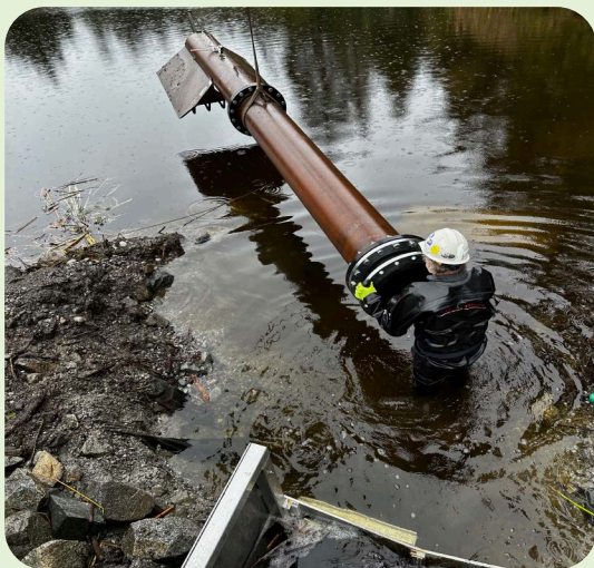
Jim Wilson in his dry suit positioning the pipe. Note the "oven-hood" end that prevents the beaver from blocking the bottom-positioned intake with mud, trees, sticks, etc.
